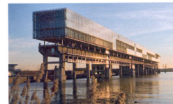
Kraanspoor, office building in Amsterdam-North Architekten: OTH, Amsterdam
